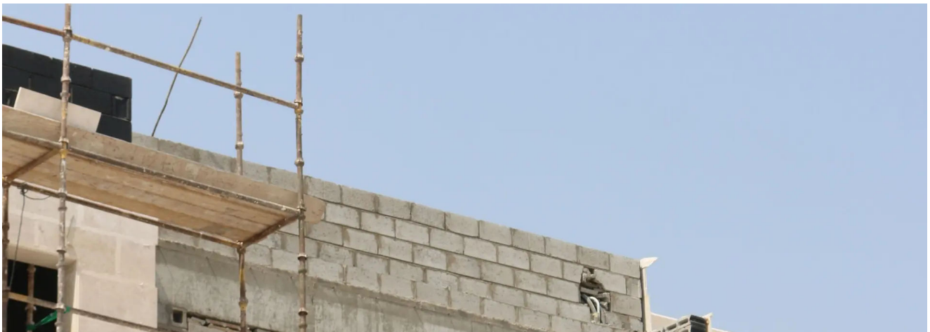
Stone facade under construction, Doha.
